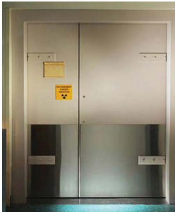
Lead-Lined Double Door with Stainless Steel Protection Panel
